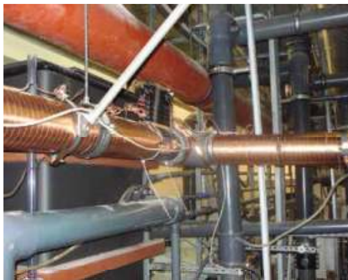
Vulcan S250 treating main water pipes for the Meridan Pool and Spa area
