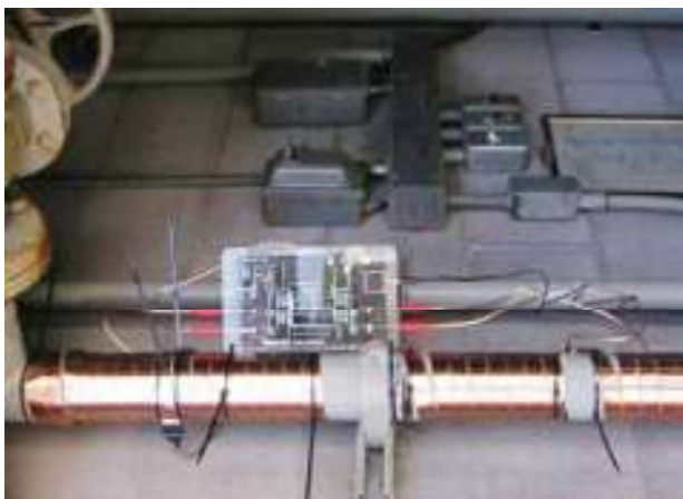
Vulcan S25 installed on cold water pipe for the Bodega marine laboratory
