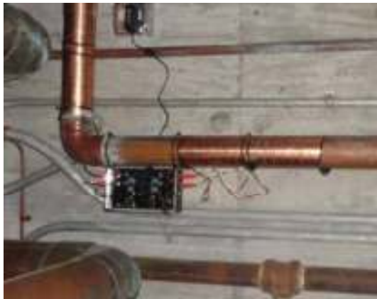
Vulcan unit installed on water main
