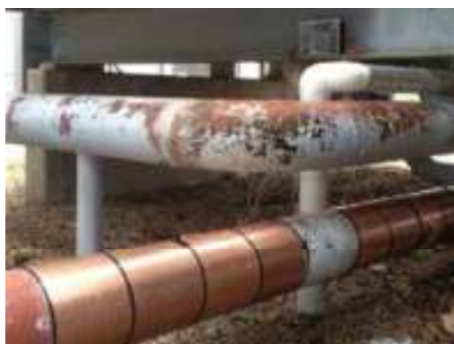
Vulcan S250 installed on a 10 inch diameter line that feeds twin cooling towers (CT-1 and CT-2)
