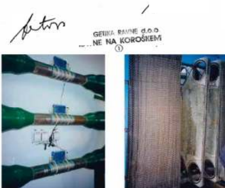
Control of honey comb fill of cooling tower
