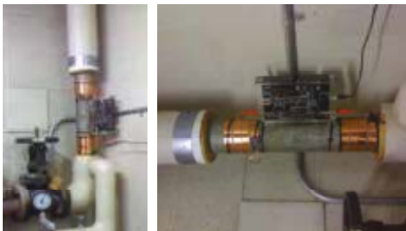
Installation of Vulcan Descaler for the entire building's water supply in the Roosevelt school
