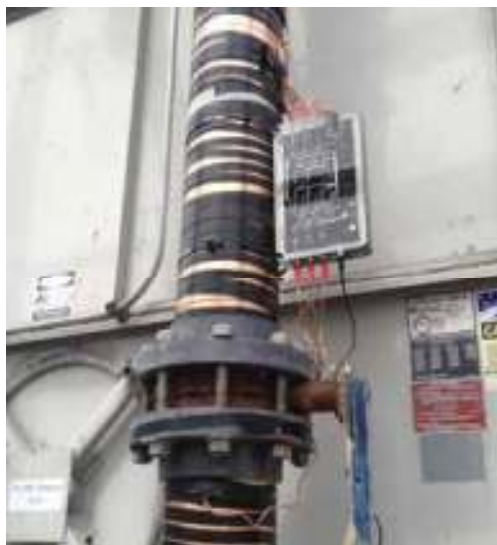
Vulcan S100 installed on cooling towers
